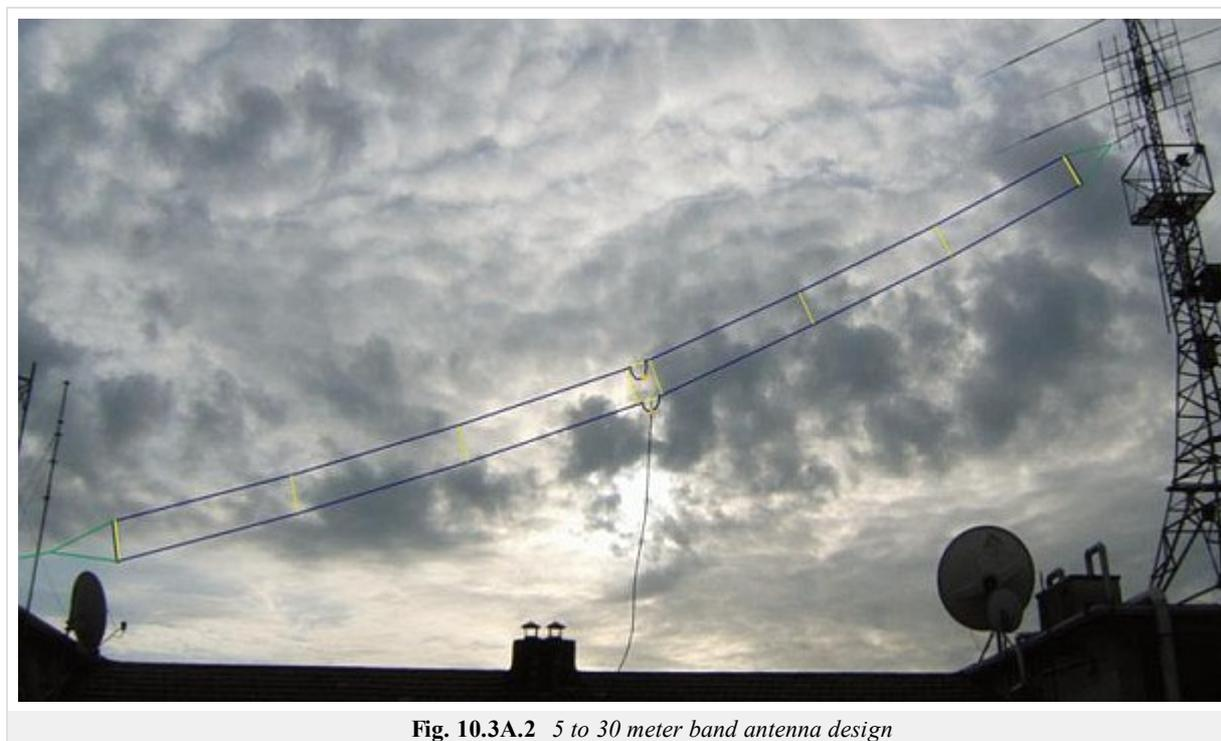
A typical T2FD is built as follows, out of two parallel wire conductors:
